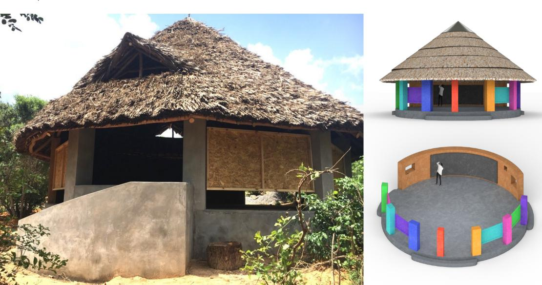
The roof is made from palm leaves. This is great for keeping the space cool and also when it rains, it does not make a lot of noice - unlike the classrooms we have with tin sheet roofing.
