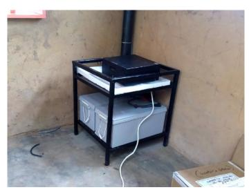
3 solar panels were attached to the roof and connected to the inverter and two batteries that are placed inside the room. Next step is to get tanks to collect the rainwater.
