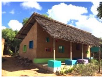
We removed the thatched roof, put in iron poles and made the roof higher adding tinn sheets and some transparent ones to let in light. And put thatched roof in front.
