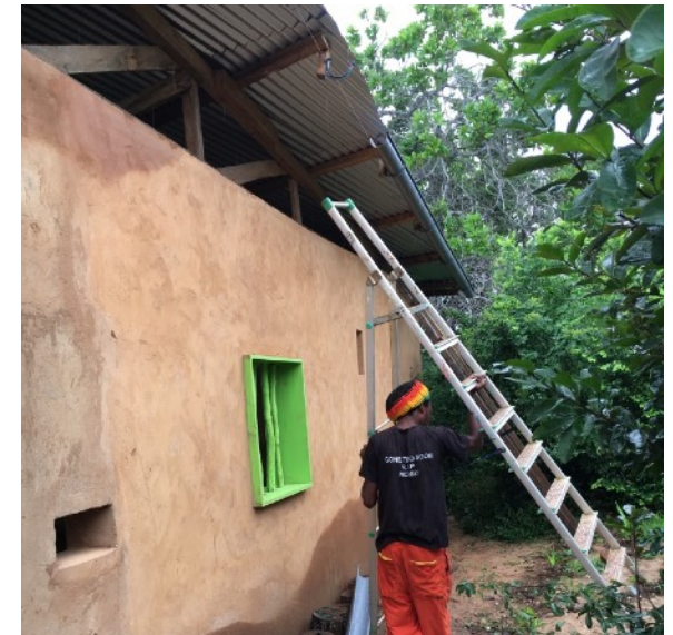
Added gutters to existing roofs to catch more water
