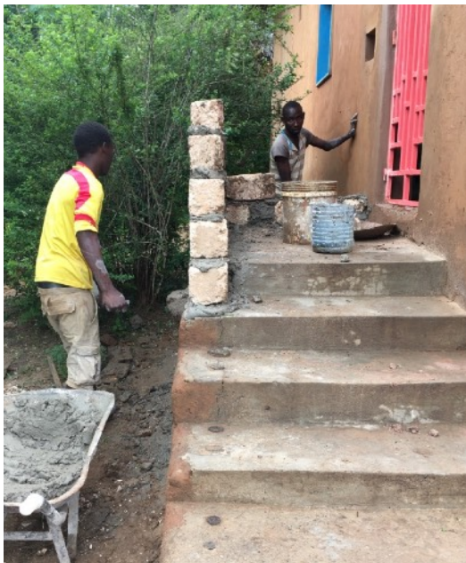
New plastering on stairs in 3 different classrooms
