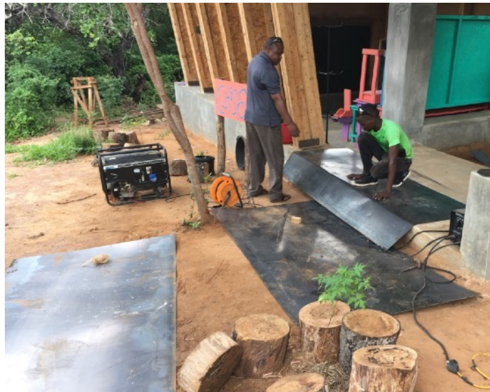
Custom made new gutters for class 3 and 6
