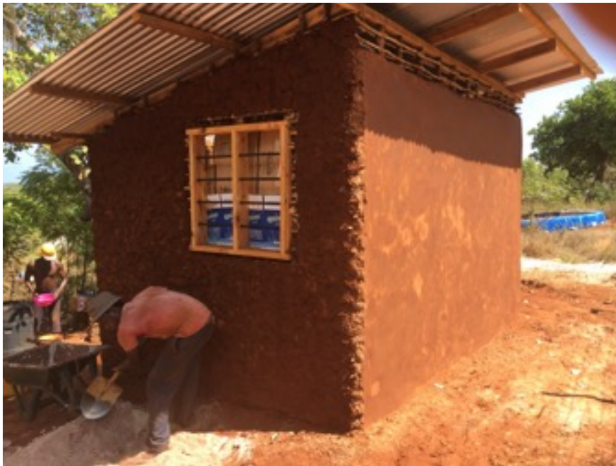
Plastering of our house and the security house using only mud and sand (local style)
