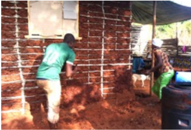
Plastering of our house and the security house using only mud and sand (local style)
