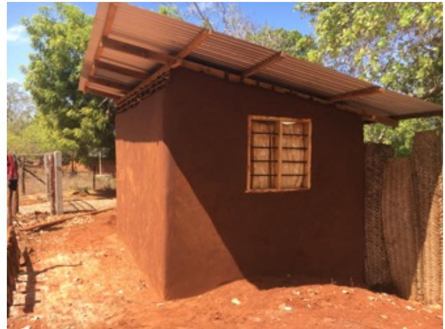
Plastering of our house and the security house using only mud and sand (local style)
