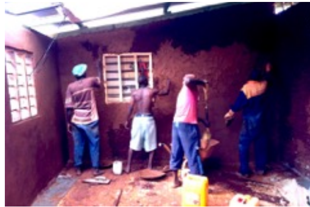
Plastering of our house and the security house using only mud and sand (local style)
